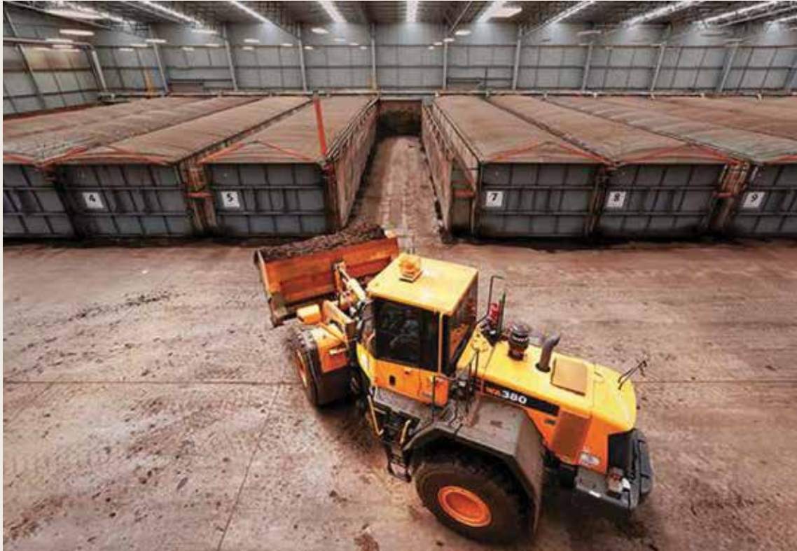
Veolia Organic In-vessel Composting Facility, Bulla Victoria.
